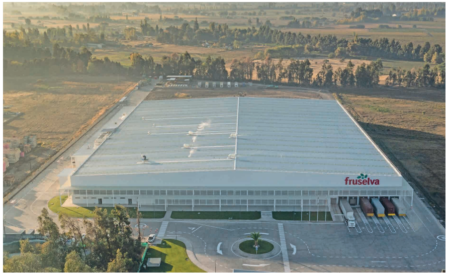
Factory in Talca, Chile / Fábrica en Talca, Chile
